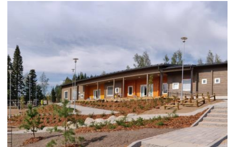
Timber day care centre
